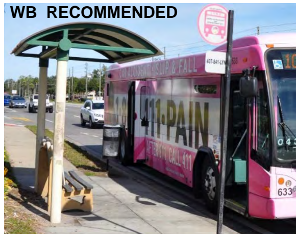
SR 50 BRT Station Analysis
